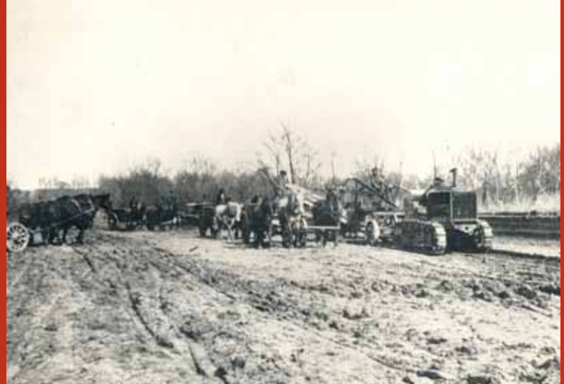
Early heavy equipment works side-by-side with teams of horses on this construction site in Herculaneum, Mo., in the early 1920s.
